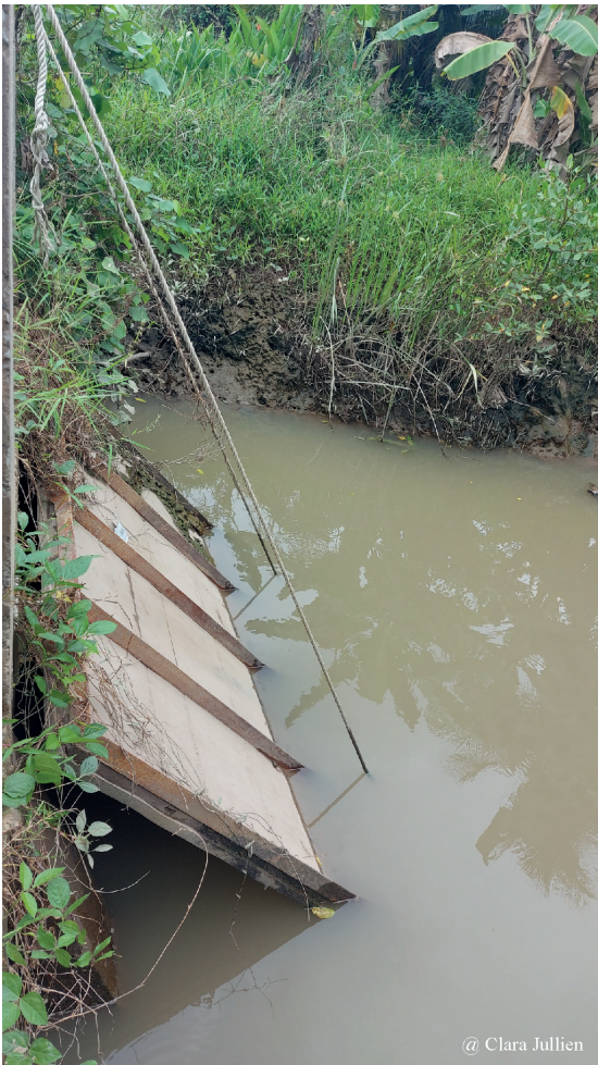
[ Figure 2/7.3 ] Failing public sluiceway in Long Dinh commune, Binh Dai district, Ben Tre province Photo credit: ©Clara Jullien - 01/04/2022
