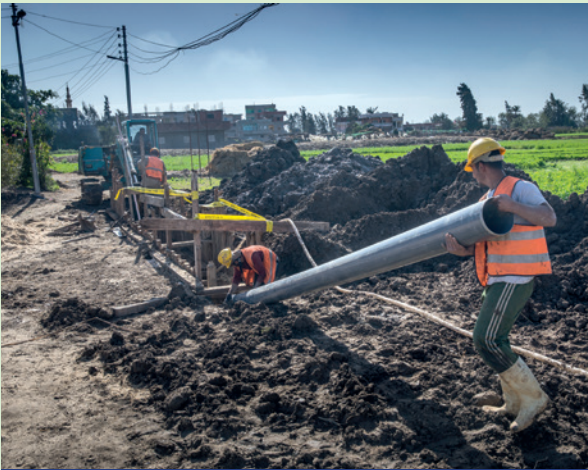
IWSP project: Installation of drinking water and sanitation pipes in the Delta in Egypt. ©AFD - KFW
