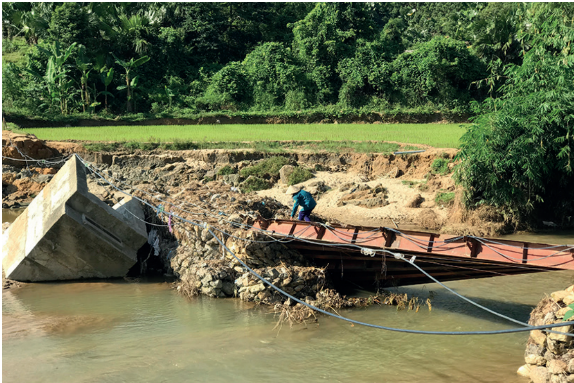
[Figure 11.4] Bridge destroyed by flash flood in November 2018
